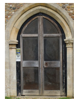
9.2.10 Limewater consolidation to south porch stonework 14.5 £500
