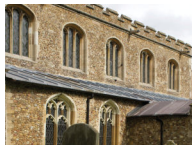
9.2.4 Repoint whole length of cover flashing at clerestory abutment to South aisle 10.6 £600
