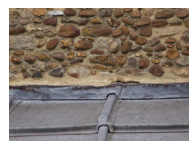
9.2.4 Repoint whole length of cover flashing at clerestory abutment to South aisle 10.6 £600
