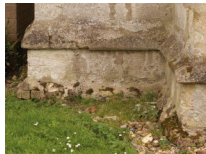
9.2.5 Minor low level repointing to Tower plinth and limewater consolidation to clunch to Tower west window 14.1 £750
